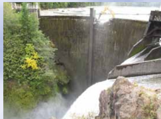
Glines Canyon Dam
