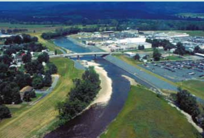
Moorewood, West Virginia, Levee
