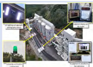
Concrete Aggregate AI Arrival Management System Prevent human errors by comparing aggregate images using AI recognition and OCR reading of incoming delivery documents
