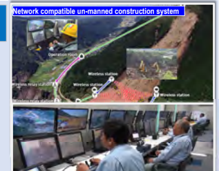
Network Style Unmanned Construction System Aso Ohashi Bridge Area Unmanned Construction Movie for ACECC Awards
