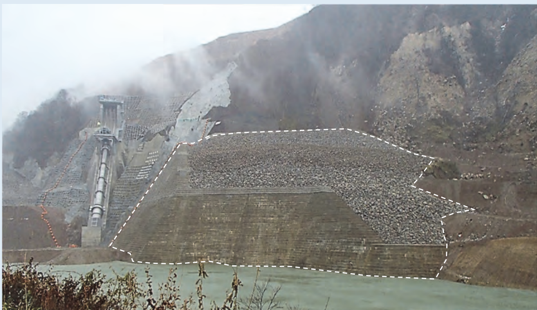
Landslide Countermeasure
