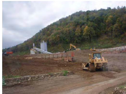
Photo-15 Secondary Stock of CSG Material
