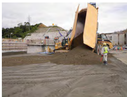
Photo-17 CSG Placing Work
