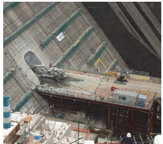
To avoid impact from vibration at the time of drilling start
