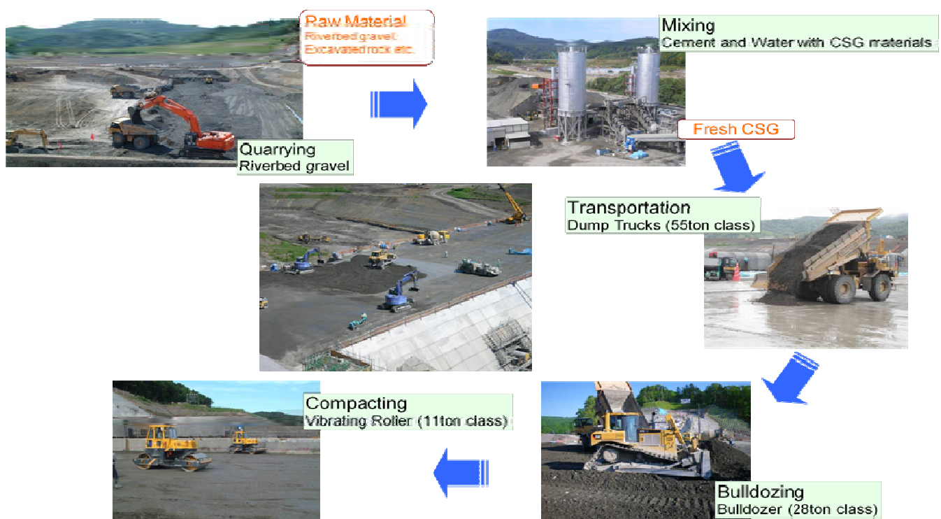
Photo-16 Construction Flow for a Trapezoidal CSG Dam
