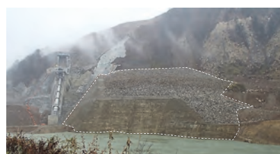
⑧ Landslide countermeasure (Isawa dam Reservoir)
