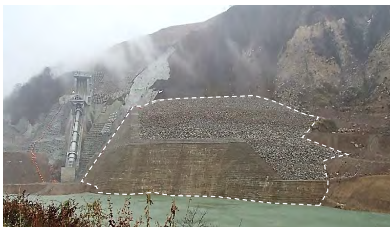
Photo-8 Landslide Countermeasure (Isawa Dam Reservoir)
