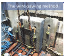
To avoid impact from vibration during penetration
