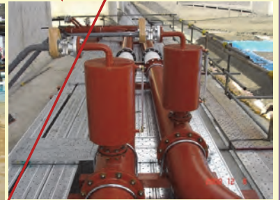
Conveyance unit - Sediment discharge pipeline & pressure regulator
