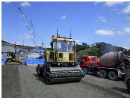
Photo-12 Control of Roller Compaction Energy (At the placing site)
