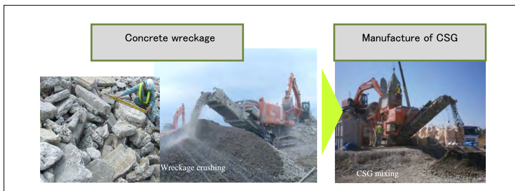
Photo-9 CSG Manufacturing Process of Small CSG Structure (Coastal Levee)
