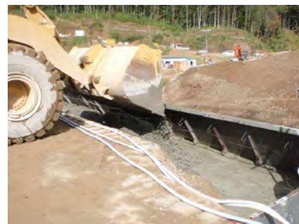
Photo-18 Protection Concrete Placing Work
