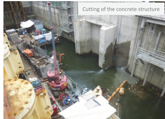
Cutting parts by wire saw under water
