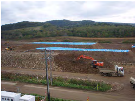
Photo-14 Primary Stock of CSG Material
