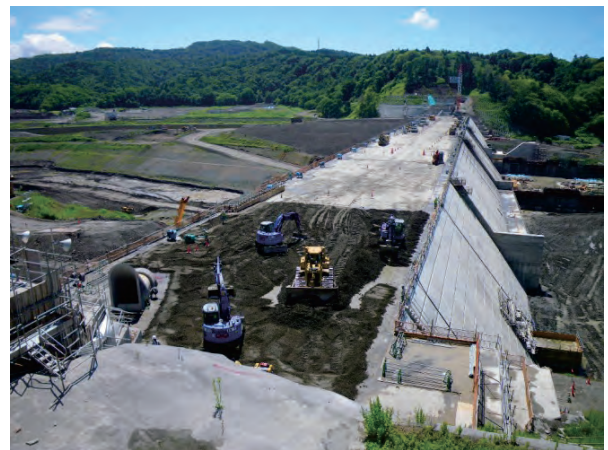
Figure-2 Tobetsu Dam
