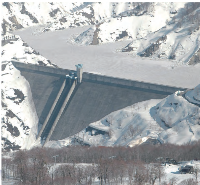
Figure-9 Okutadami Dam
