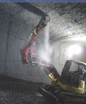
Finish drilling, improvement of drilling accuracy
