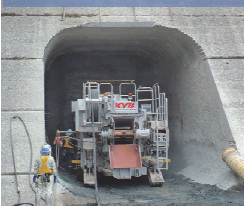
Main drilling, reduction of vibration at the time of drilling
