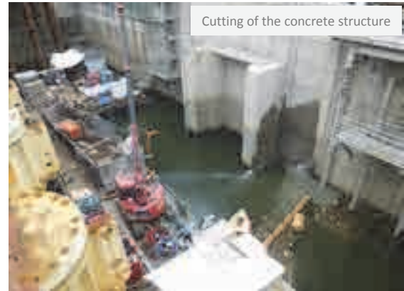
Cutting parts by wire saw under water
