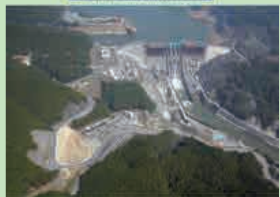
Some construction items at the end of March 2019
