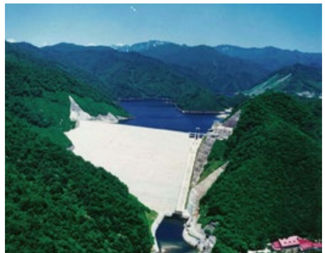
Figure-7 Naramata Dam
