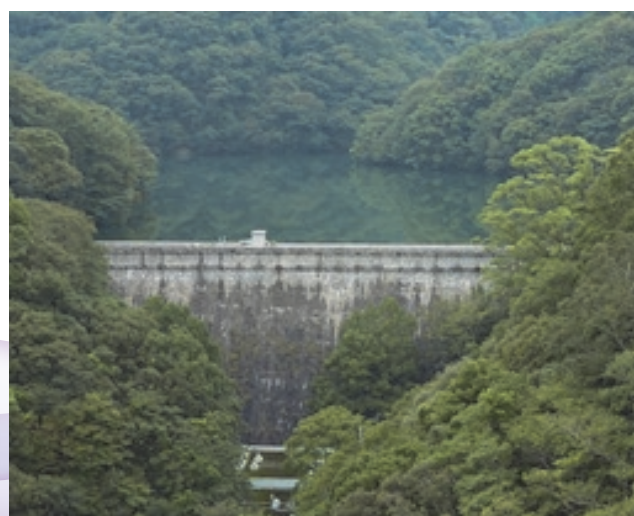
Figure-5 Nunobikigohonmatsu Dam
