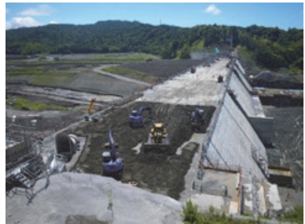
Figure-2 Tobetsu Dam
