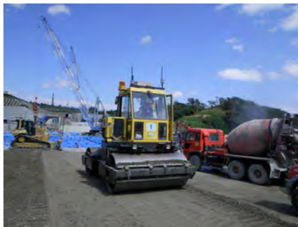
Photo-12 Control of Roller Compaction Energy (At the placing site)
