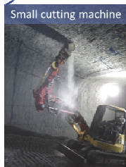
Finish drilling, improvement of drilling accuracy
