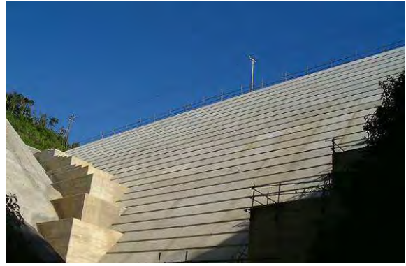
Photo-4 CSG Sub Dam (Taiho Dam)
