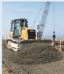
Bulldozing Bulldozer (7t class)
