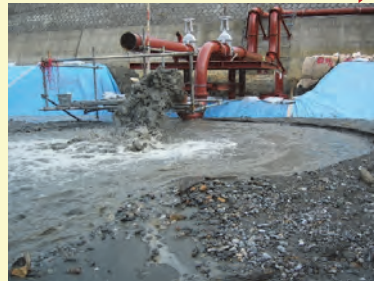
Outlet unit - View of Sediment dredging
