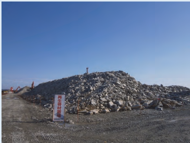
Stock Yard of Concrete Wreckage (Raw Materials of CSG)
