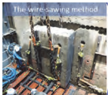
To avoid impact from vibration during penetration
