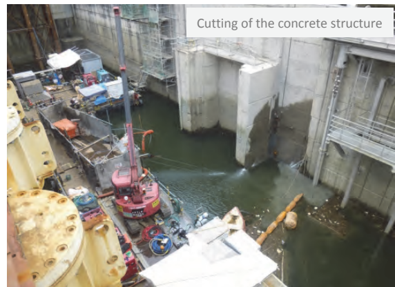
Cutting parts by wire saw under water
