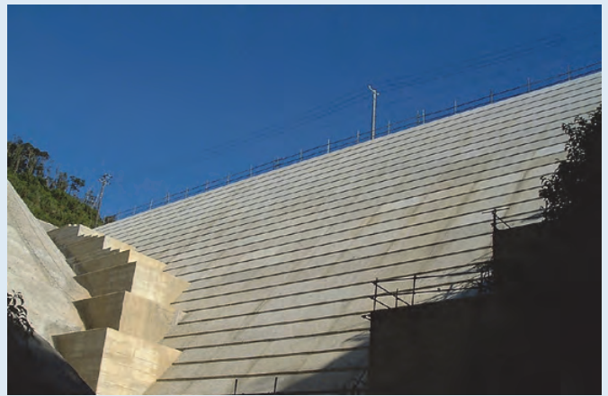
CSG Sub Dam
