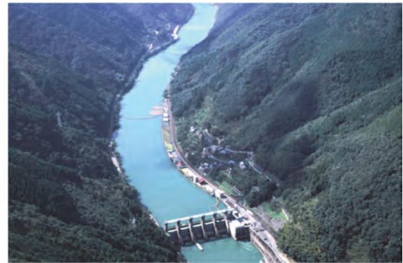
Figure 4 Setoishi Dam, Hydropower Plant and Reservoir
