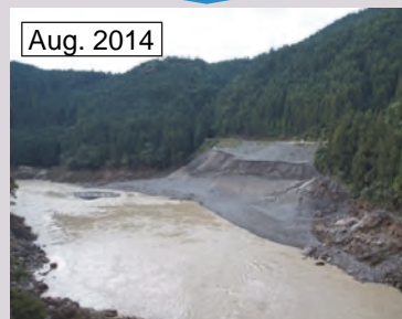
88,000m 3 sediments out of 185,000m 3 were flushed out.
