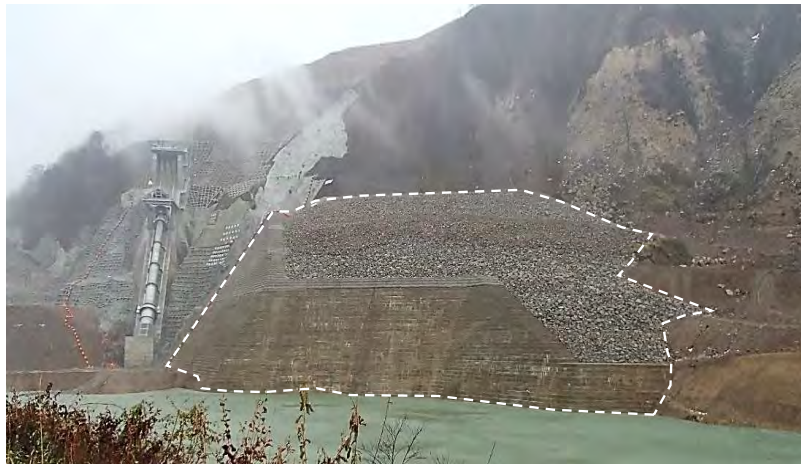
Photo-8 Landslide Countermeasure (Isawa Dam Reservoir)
