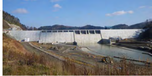
③ Sanru Dam
