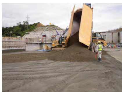
Photo-17 CSG Placing Work
