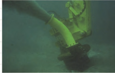
Sand pump suctioning
