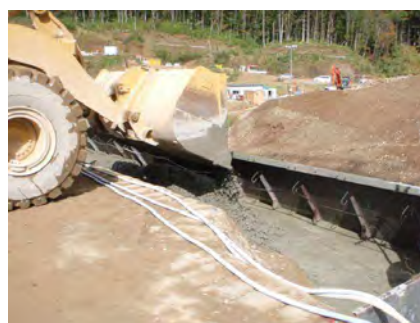
Photo-18 Protection Concrete Placing Work
