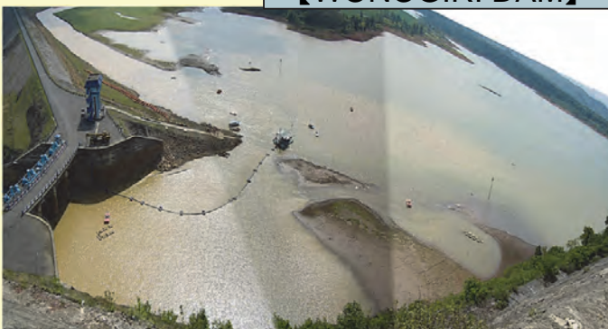
View of dredging site
