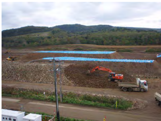
Photo-14 Primary Stock of CSG Material
