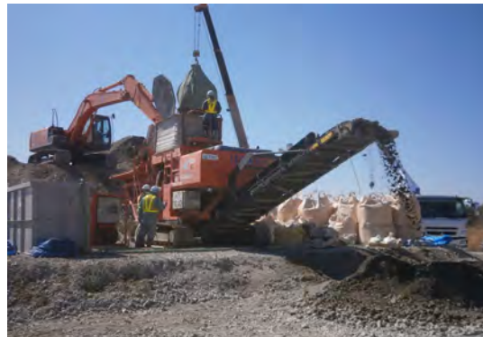
Mobile Soil Remediation Machine (For Small structure; Natsui Coastal Levee)
