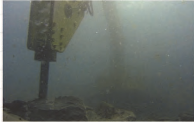
Rock crushing with a breaker
