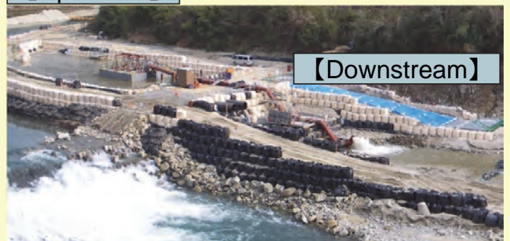
View of siphon dredging facility
