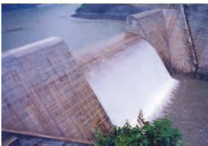
⑦ Nagashima Sediment Check Dam
