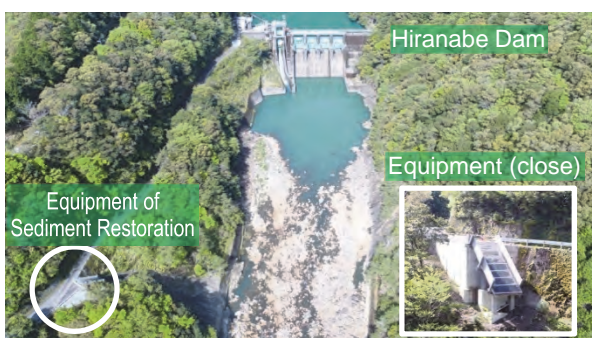
Figure 2 Equipment of Sediment Restoration
