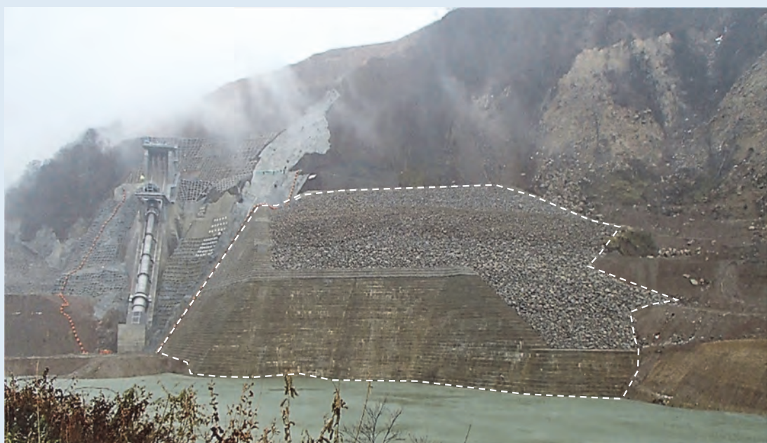
Landslide Countermeasure
