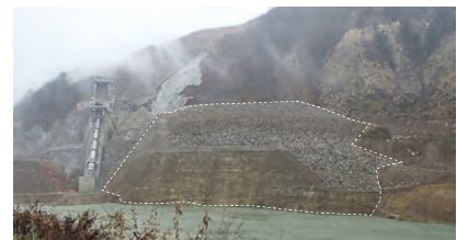
⑧ Landslide countermeasure (Isawa dam Reservoir)
