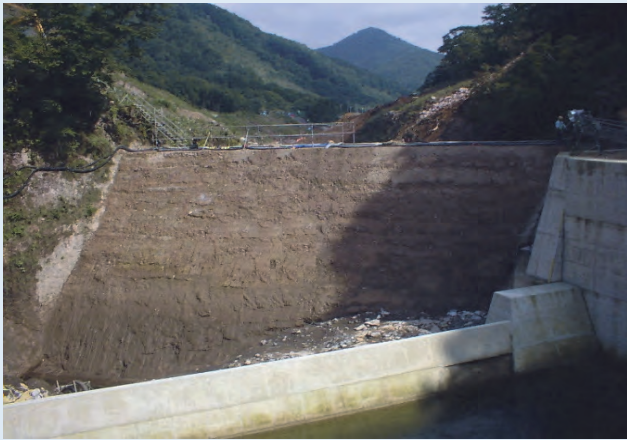
CSG Sediment Check Dam
