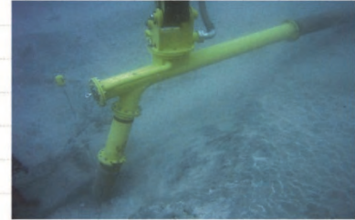
Cleaning by an ejector
