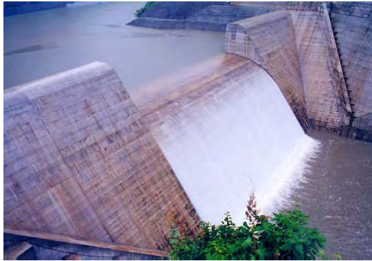
Photo-3 CSG Sediment Check Dam (Nagashima Dam Reservoir)
