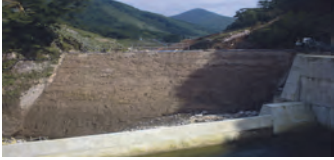
⑤ Taiho Sub Dam
