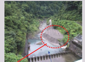
Replenished sediments by temporary placing them
