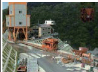
Bunker line (batcher plant)
