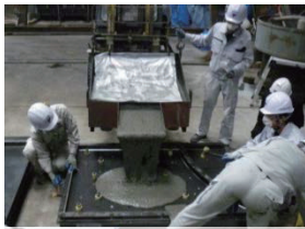
Production of the pre-cast material
