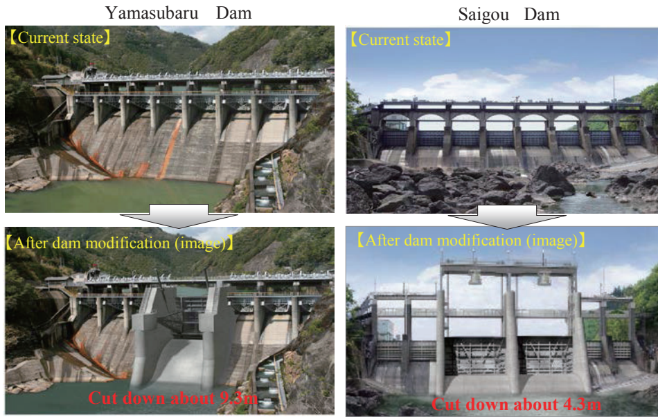
Fig2. Dam Retrofitting - Image (Yamasubaru and Saigou Dams)
