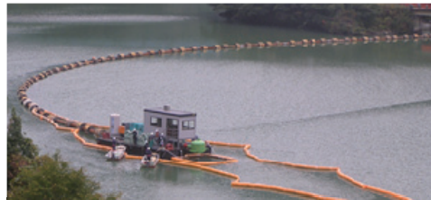
Transportation in the reservoir (Pipeline)
