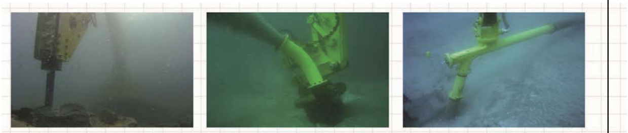
Rock crushing with a breaker
