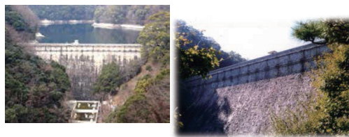
Dam (frost attack)
