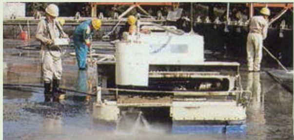
Cutting by wireless remote control
