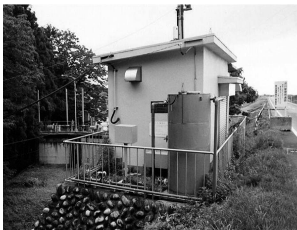
Photo 4 Real-time suspended sediment densitometer
