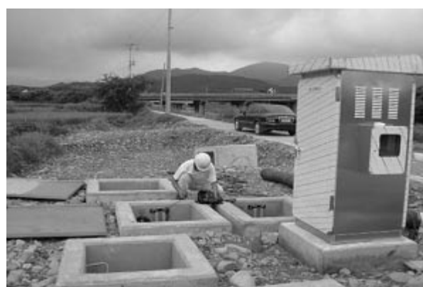
Figure 5 Installation of sewage pump
