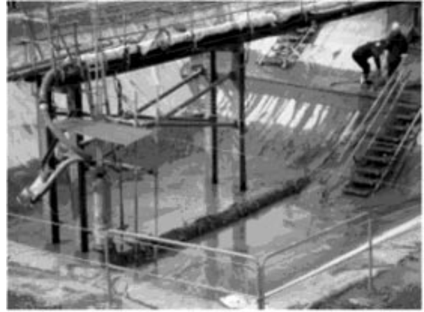
Picture-6 Geometry change of silt bed after suction
