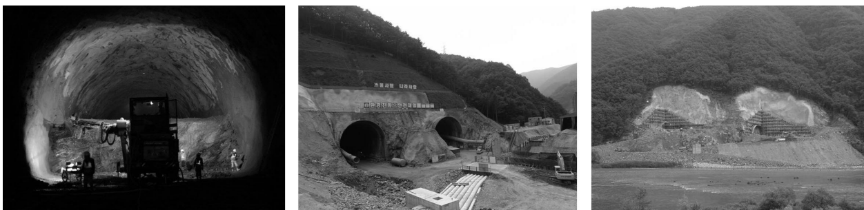
Fig. 16 Split excavation, downward tunnel portal, exit section
