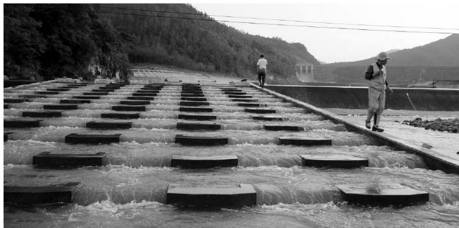
Fig. 5 One of the Pool type Ice-harbor fishway constructed in downstream of the Tamjin Dam
