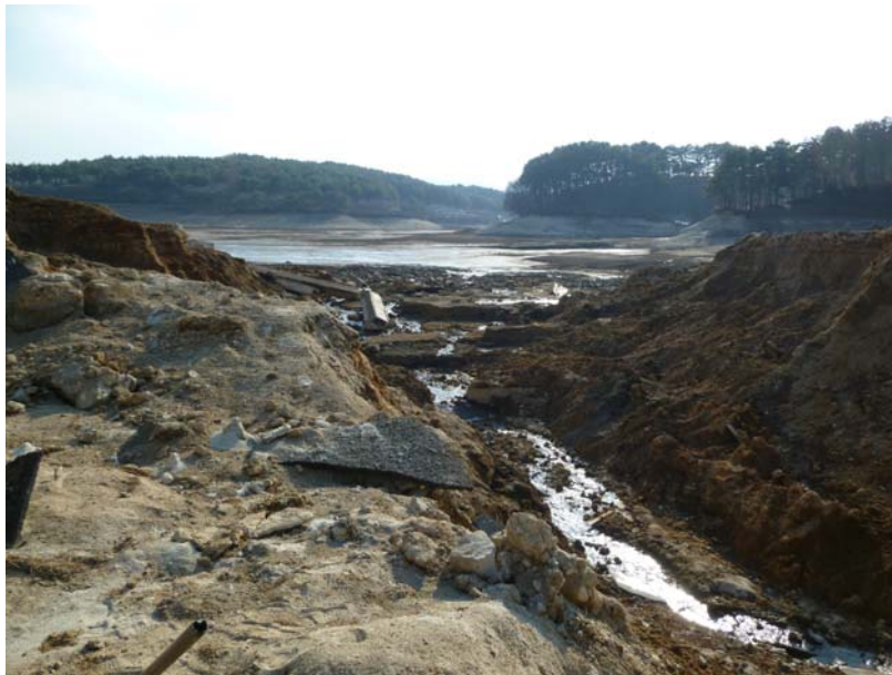
Figure 13. View from downstream toward the Fujinuma-ike
