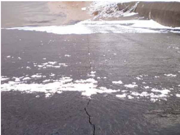
Figure 7 Asphaltic concrete face of Minamikawa Saddle Dam
