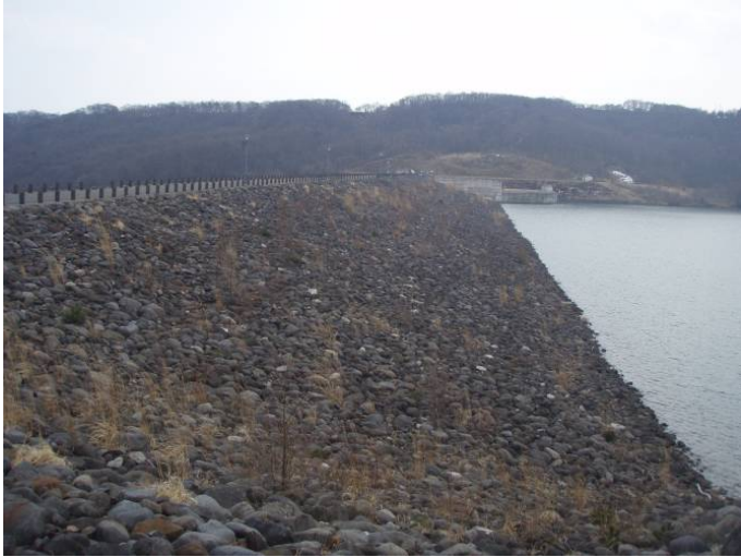
Figure 9. View of Hokkawa dam from left abutment towards right abutment
