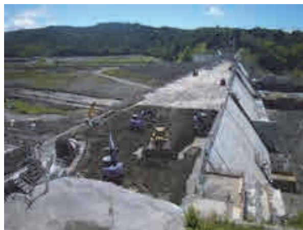
Figure-2 Tobetsu Dam
