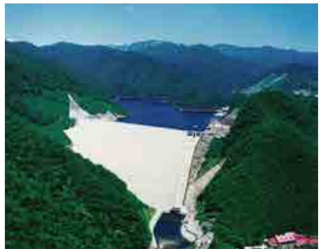
Figure-7 Naramata Dam
