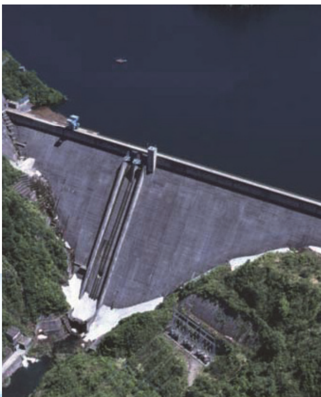
Figure-9 Okutadami Dam
