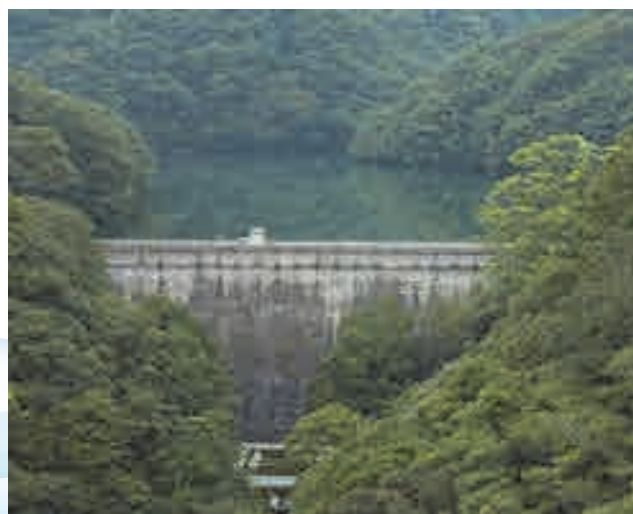
Figure-5 Nunobikigohonmatsu Dam
