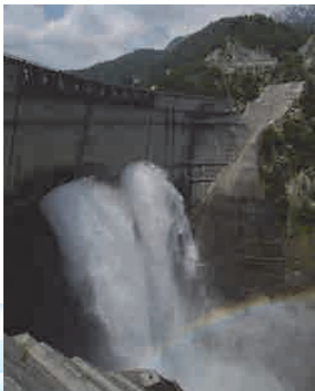
Figure-10 Kurobe Dam
