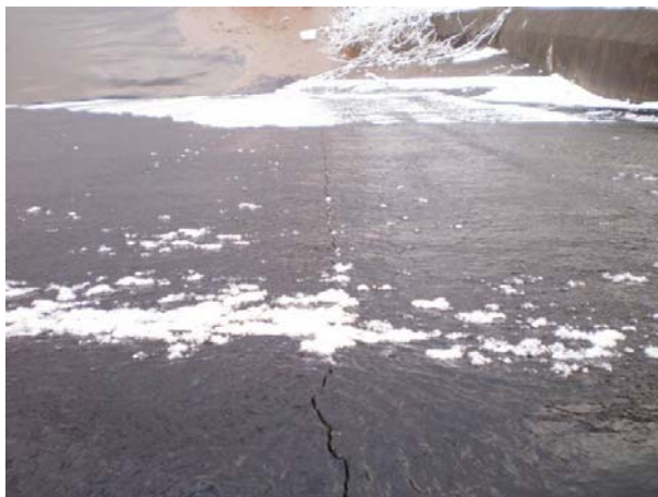
Figure 7 Asphaltic concrete face of Minamikawa Saddle Dam
