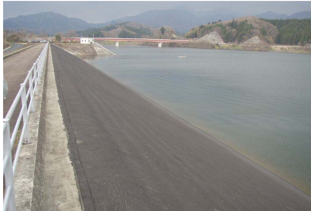
Saddle dam: asphalt concrete face rockfill
