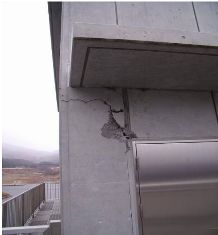
Figure 5. Cracking at gate house
