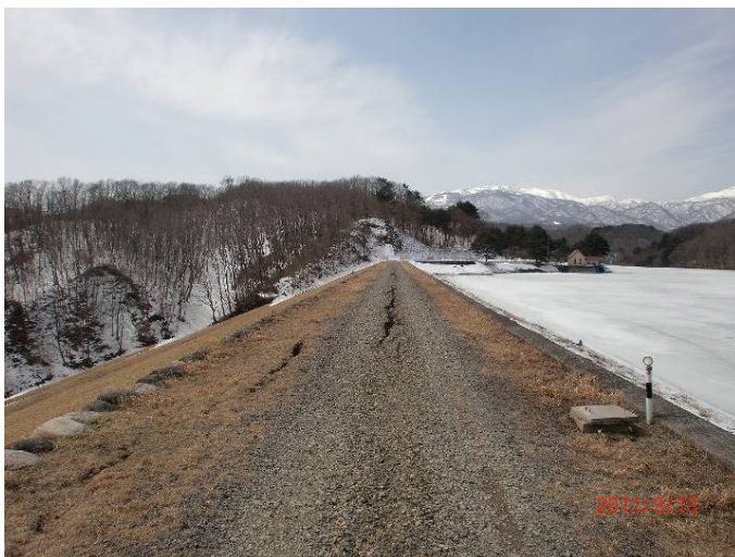
Figure 11. Nishigo Dam; cracking on the crest
