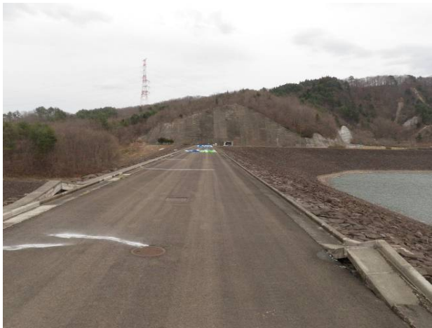
Figure 6. Bump on the crest of Nanakita Dam
